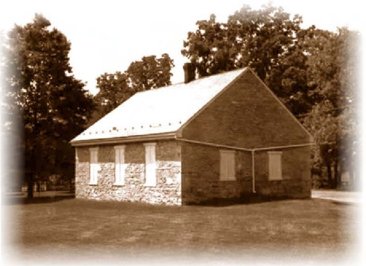
Old Brown's Mill School, Franklin County
